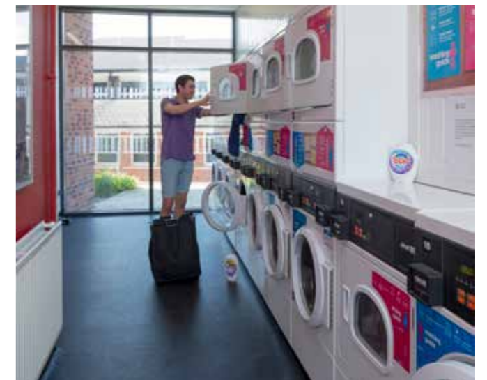
Shared laundry facilities
